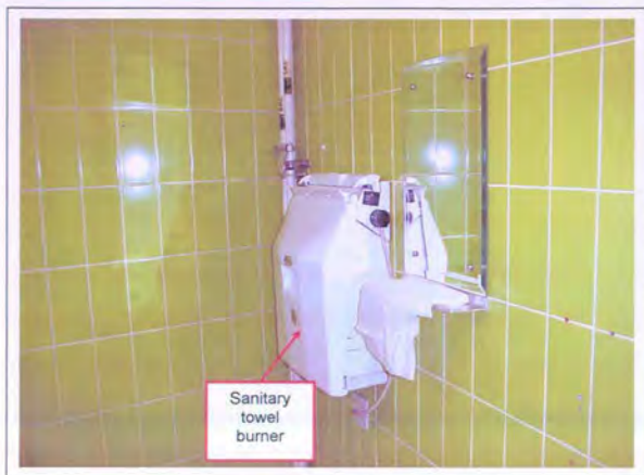
Figure 18: Material Strongly presumed To Contain Asbestos
