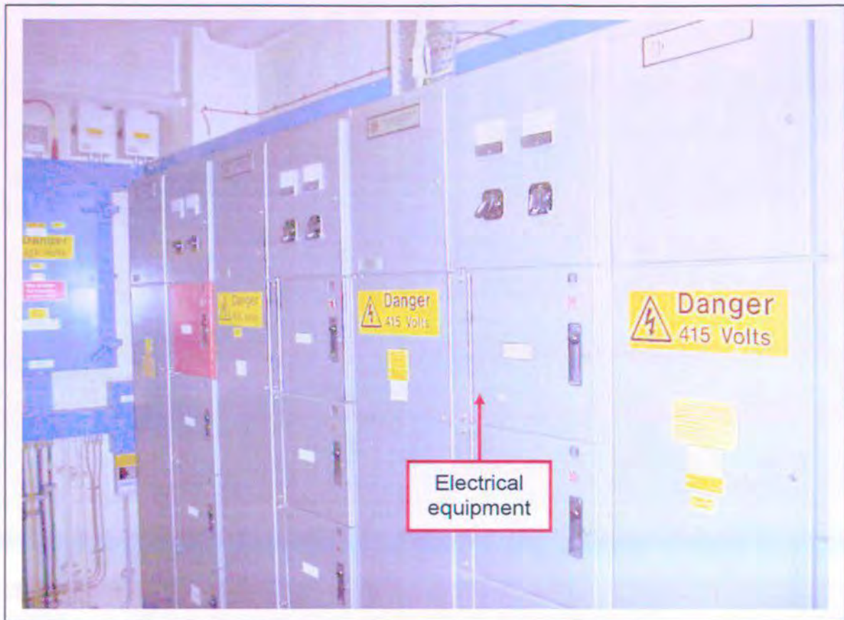
Figure 11: Material Strongly presumed To Contain Asbestos
